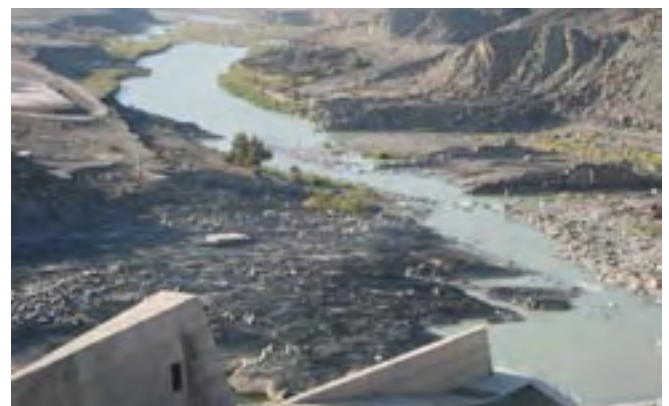
Figure 2. Pishin Dam Pond is the most important and suitable habitat for C. palustris on the Sarbaz River. Photograph: Elham Abtin.
